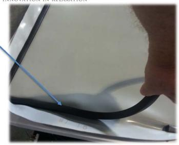
Step 5: Lay the new rubber barrier squarely in place and align with the corners of the tub.
